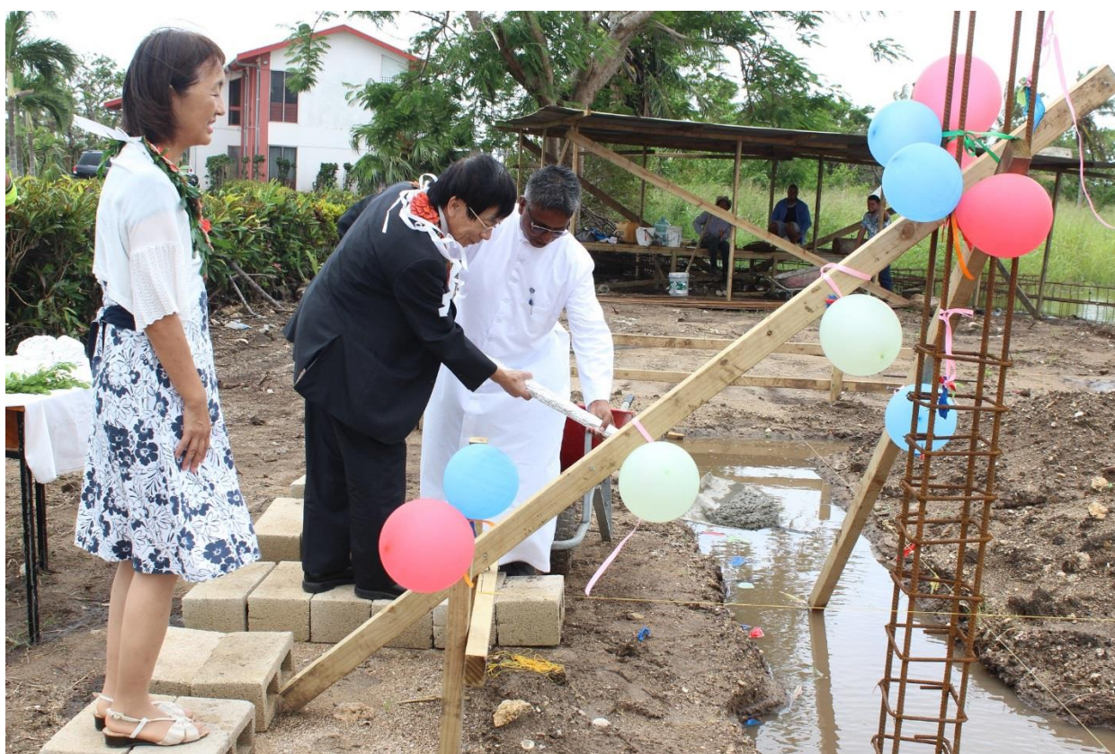
H.E Mr. Tetsuya Ishii, Ambassador of Japan to Tonga in the ground breaking ceremony to commence the construction of a student's dormitory for Montfort Technical Institute on Wednesday, 4 April 2018.
