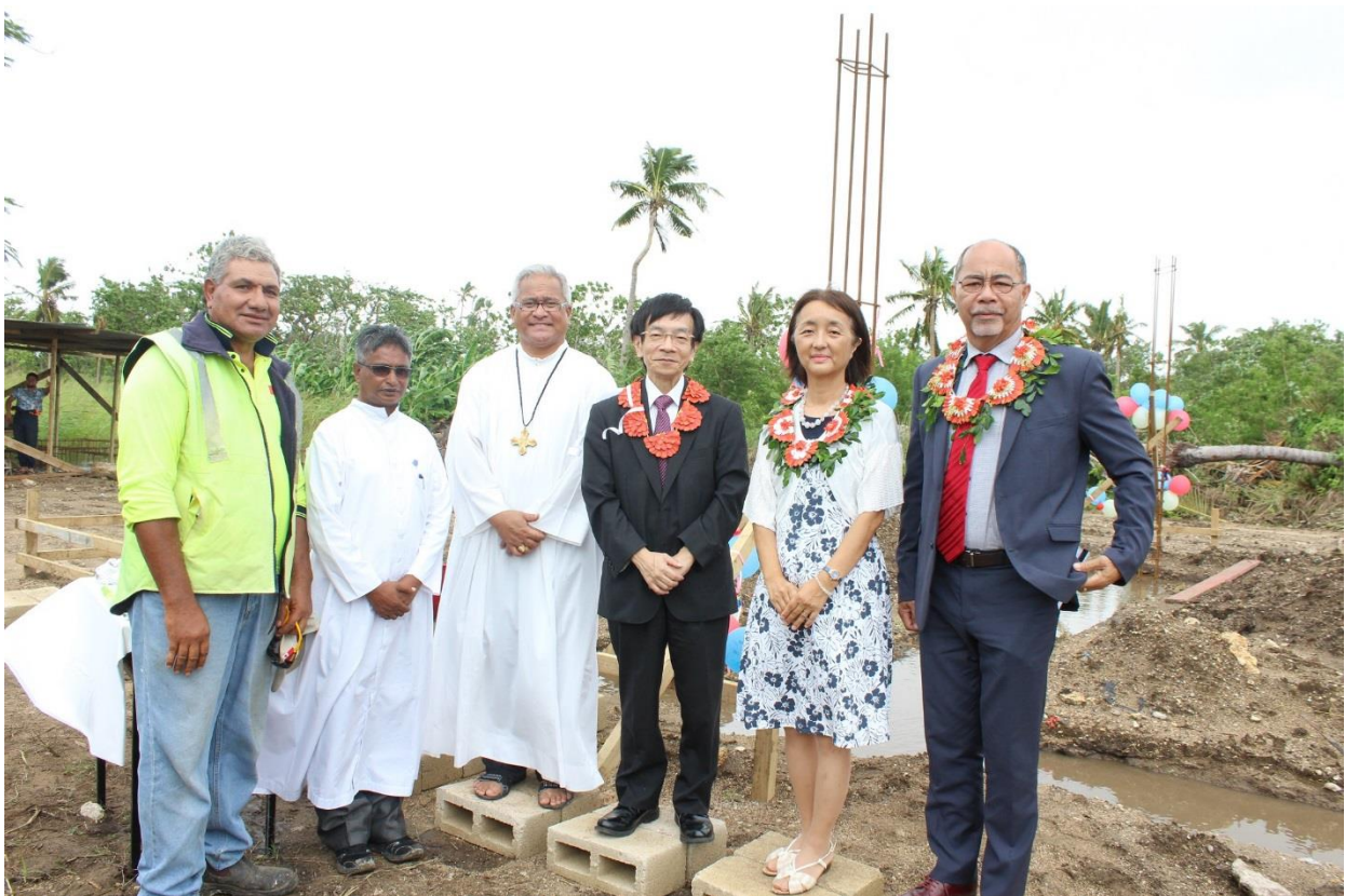
H.E Mr. Tetsuya Ishii along with Mrs. Ishii, Cardinal Mafi, Bro. Curzmeccias Sebastian with Mr. Stan Tu'amoheloa at the construction site for the new student's dormitory for Montfort Technical Institute.
