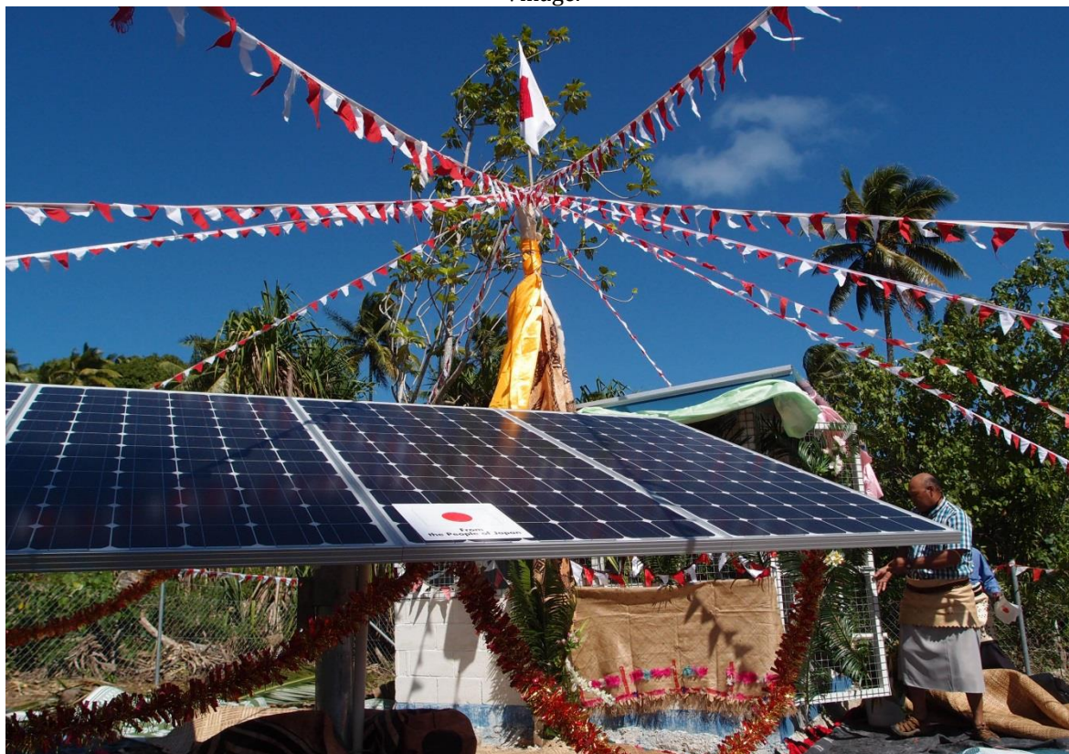
Upgraded Hihifo Water Supply Facility with solar pump systems
