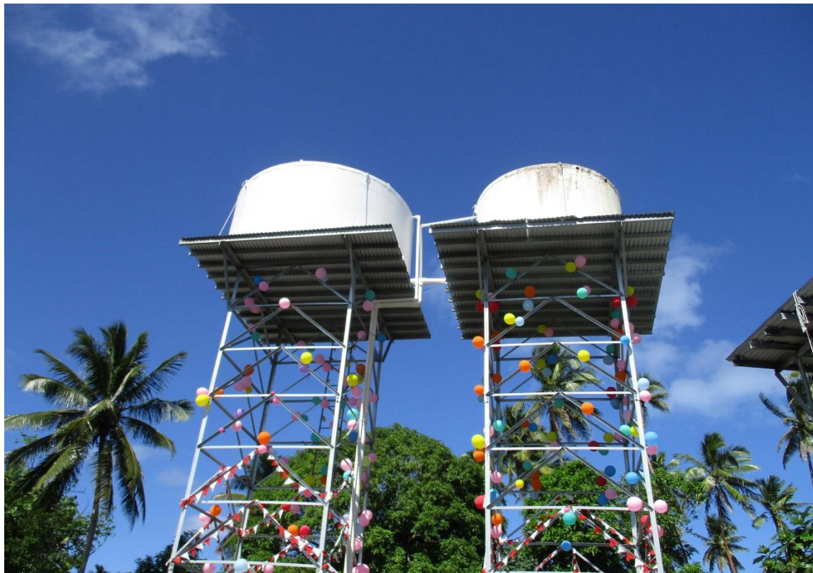
Upgraded Water Supply System for Falehau Village, in Niuatoputapu.
