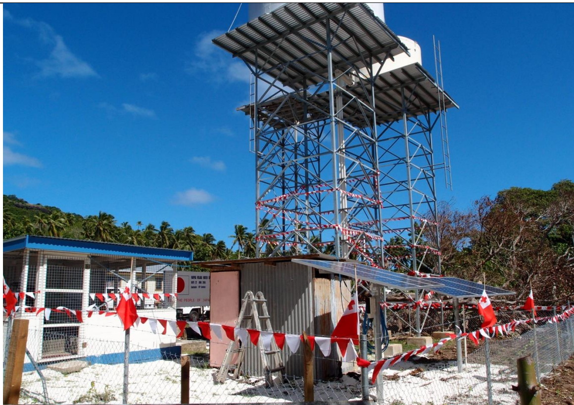
Upgraded Water Supply System for Vaipoa Village, Niuatopotapu.
