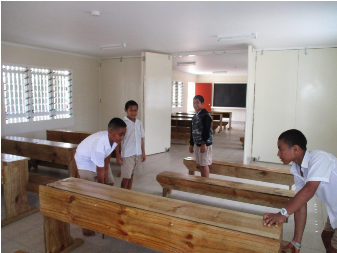
The new classroom with a partition wall and equipped with cyclone shutters
