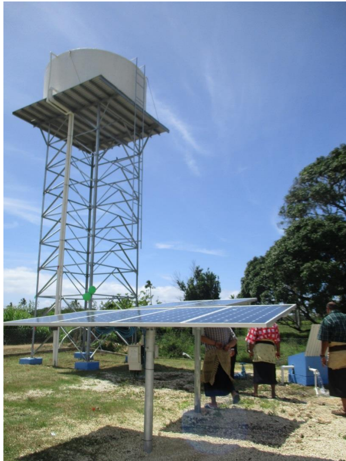
New water system with solar pump unit installed for Navutoka Village.
