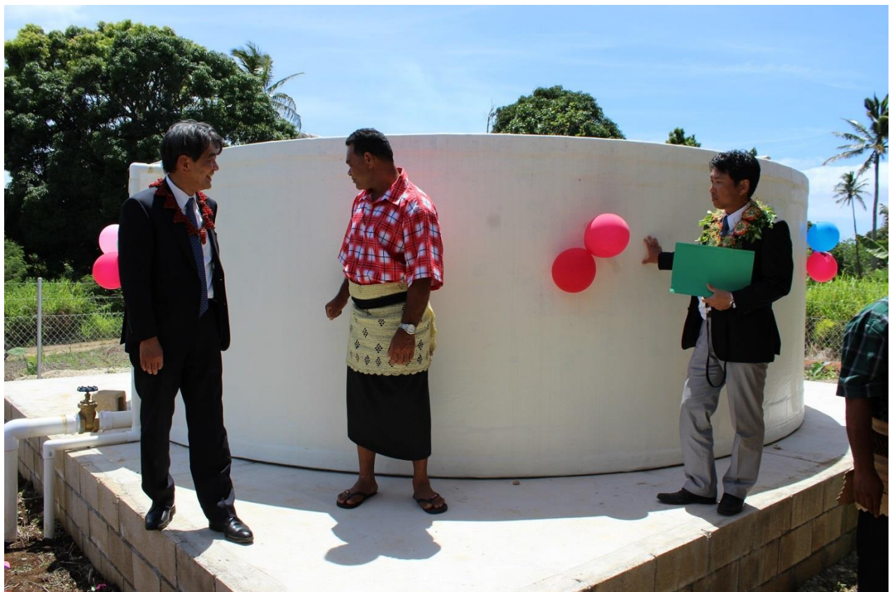
New water tank installed for Navutoka Village.
