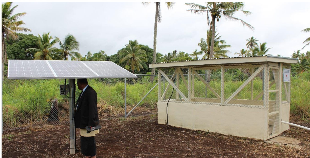
New Solar panel and pump house facility for Nukuleka Village.
