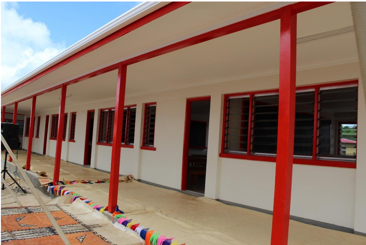
The new classroom building for Upper Room Primary School, funded through Japan's GGP Projects.
