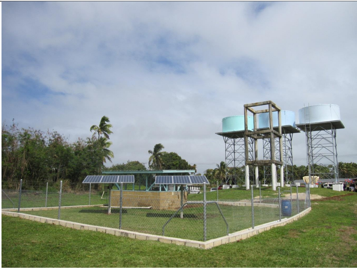
Tatakamotonga New Water Pump System
