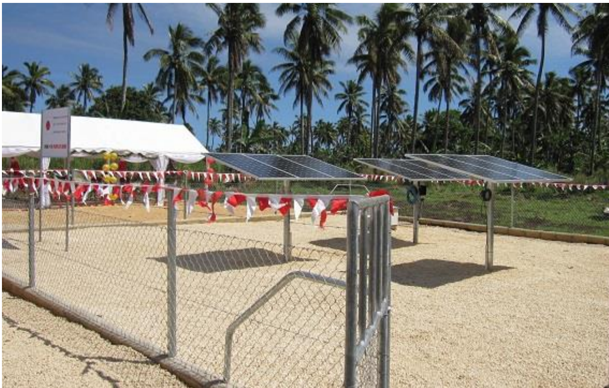
Japan's GGP funded installation of a new solar power water pump for Folaha village water supply system.
