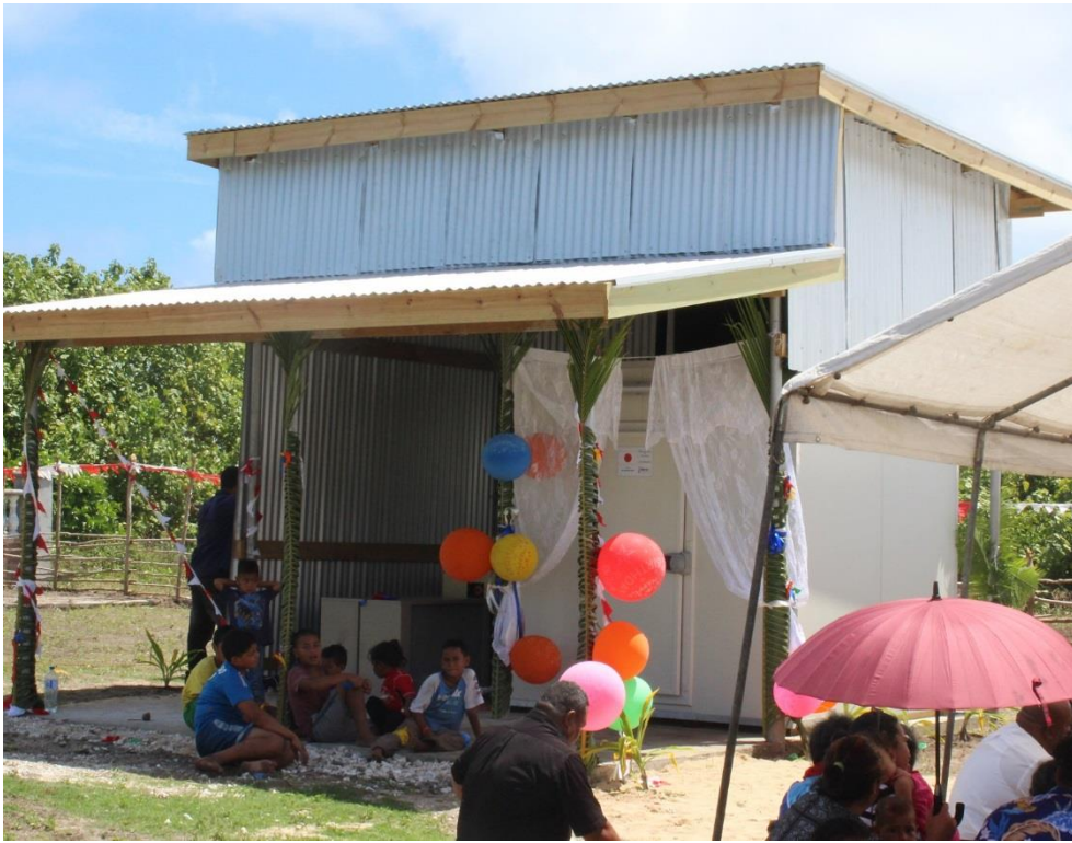
The new ice-machine system installed in 'Uiha under the funds from Japan's GGP.
