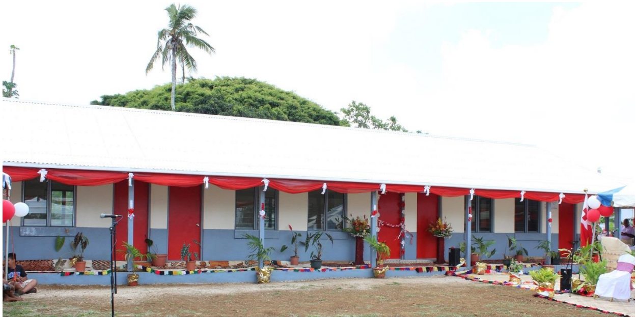
New classroom building for GPS Havelu/Tofoa
