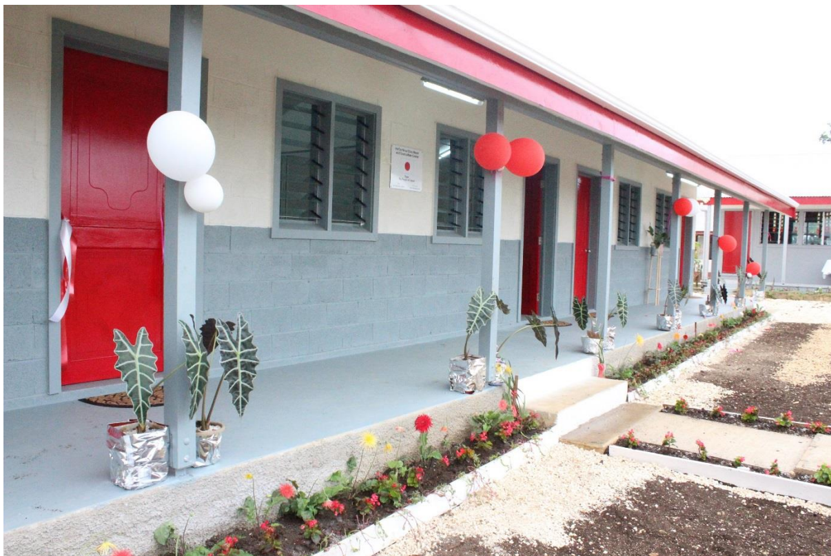
The new classroom building for Hofoa GPS.
