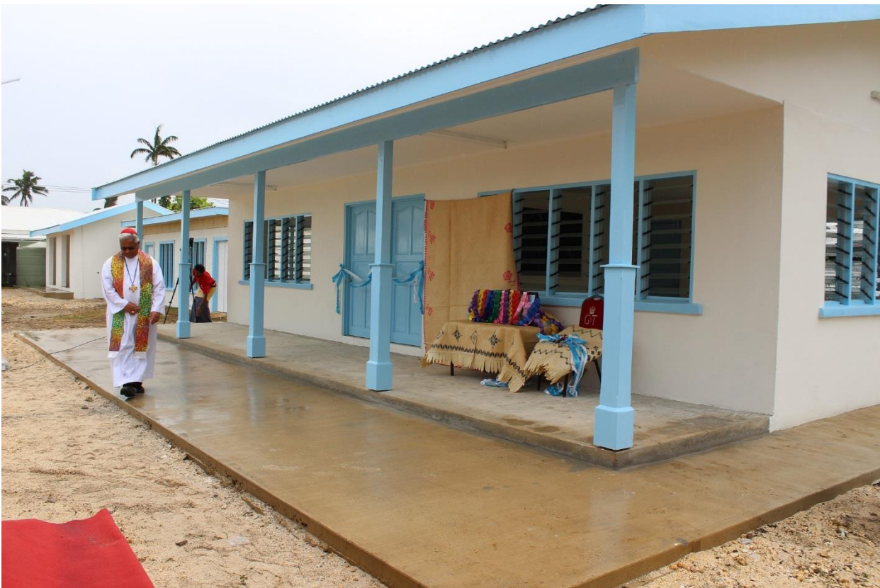
The new classroom facility funded under Japan's GGP.
