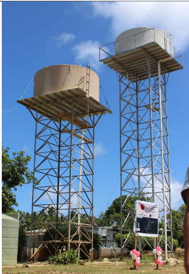
An additional tank stand (14m) with 5000 gallon water tank installed under Japan's GGP for Ha'asini and Hamula village.
