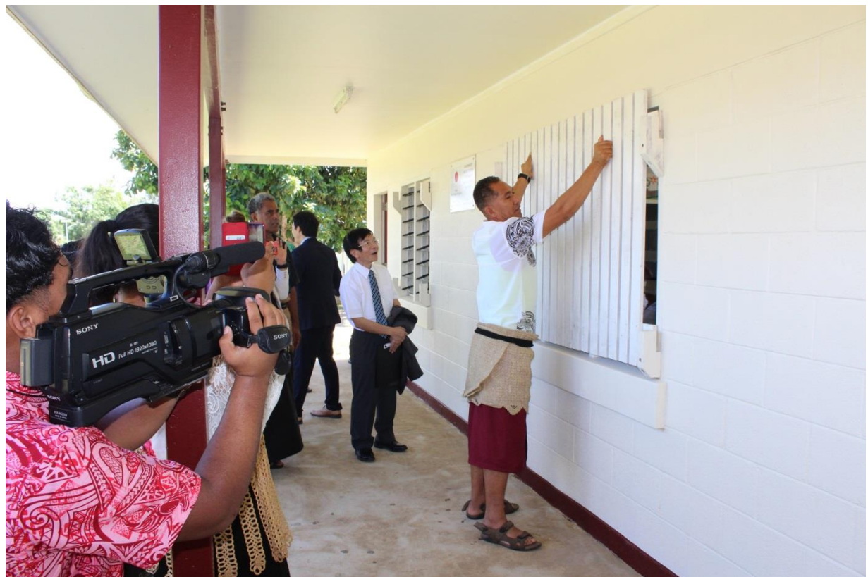
Cyclone Shelters which protected the windows from the Cyclone Gita last February.
