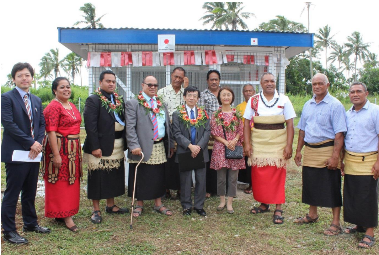
The new pump house and new water pump machine funded by the GGP Project for Talafo'ou Village.
