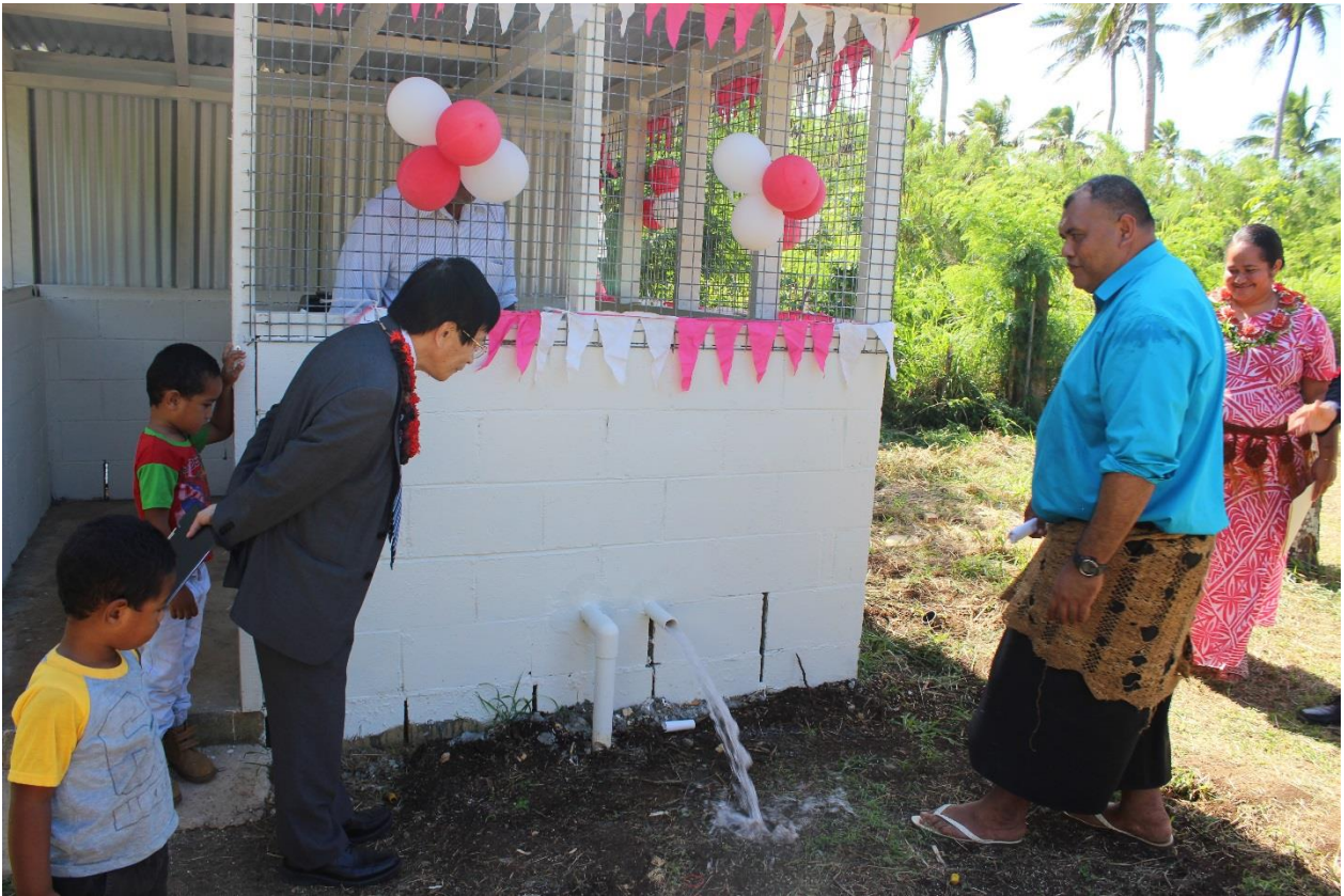
A new pump house with new water pump system for Lavengatonga village.
