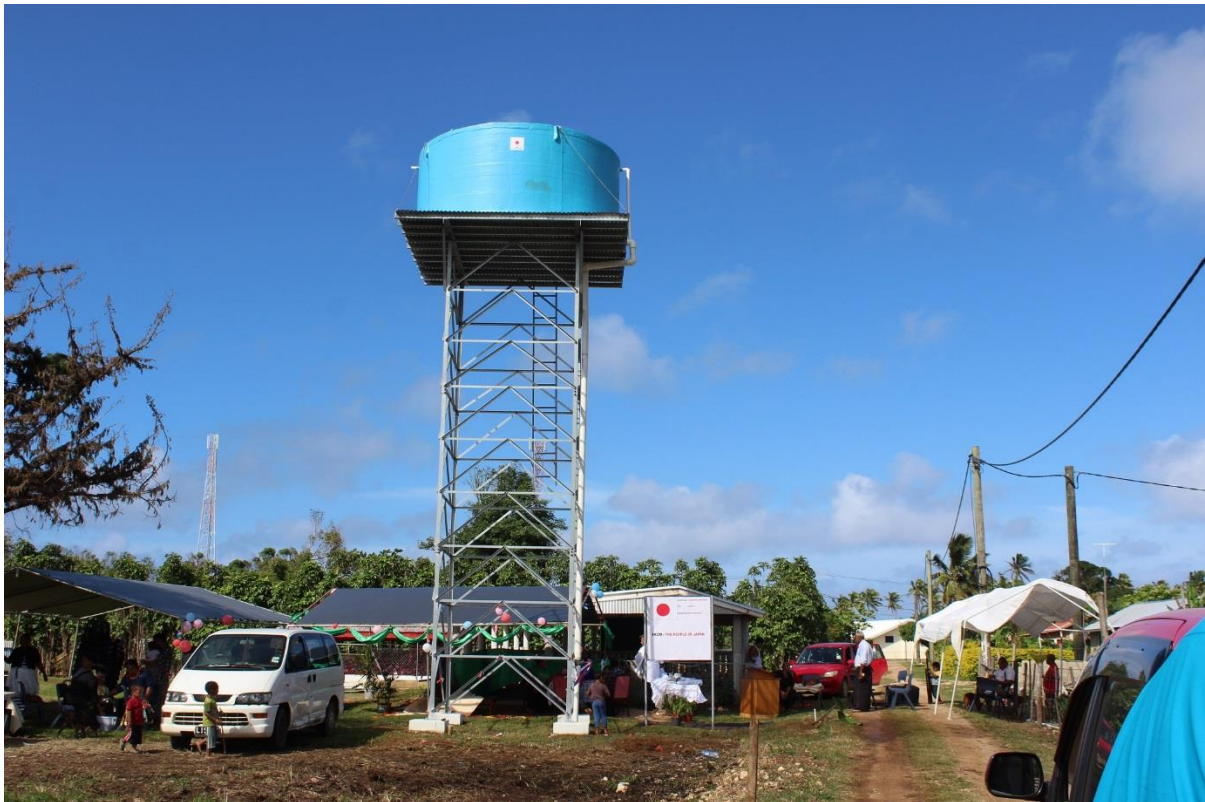
The new tank stand for Lavengatonga village, funded through Japan's GGP project.
