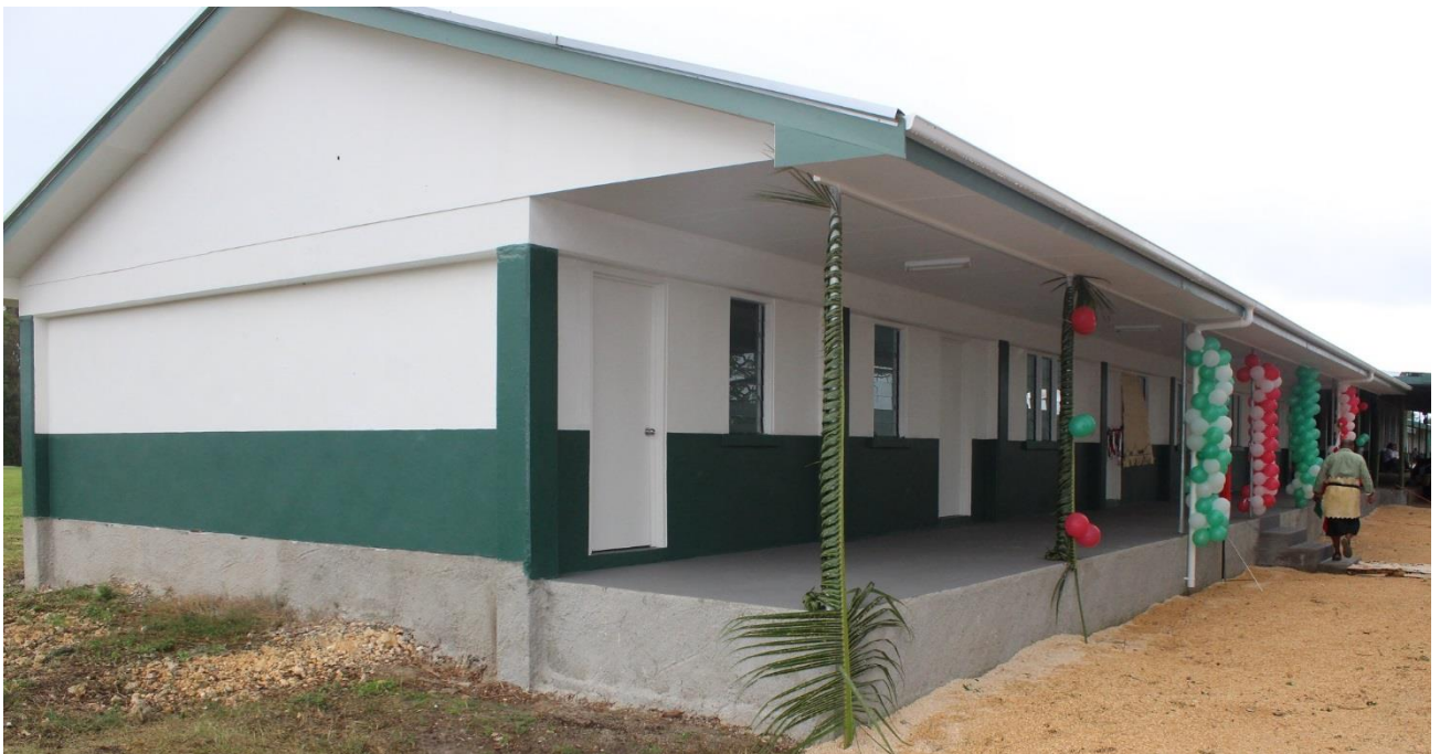
The new TVET building for Takuilau College was handed over on 8 August 2019.
