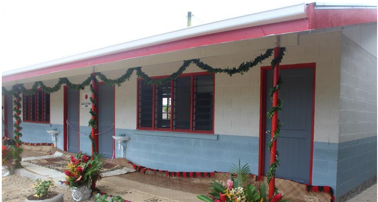
New classroom building with two rooms for Ha'alalo Government Primary School, 23 April 2020.
