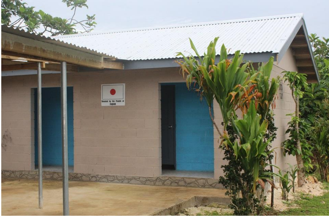
The new toilet block funded under Japan's GGP for Ha'alalo GPS.
