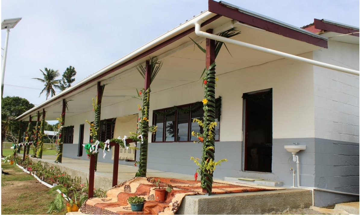
The upgraded classroom building funded by Japan's GGP.
