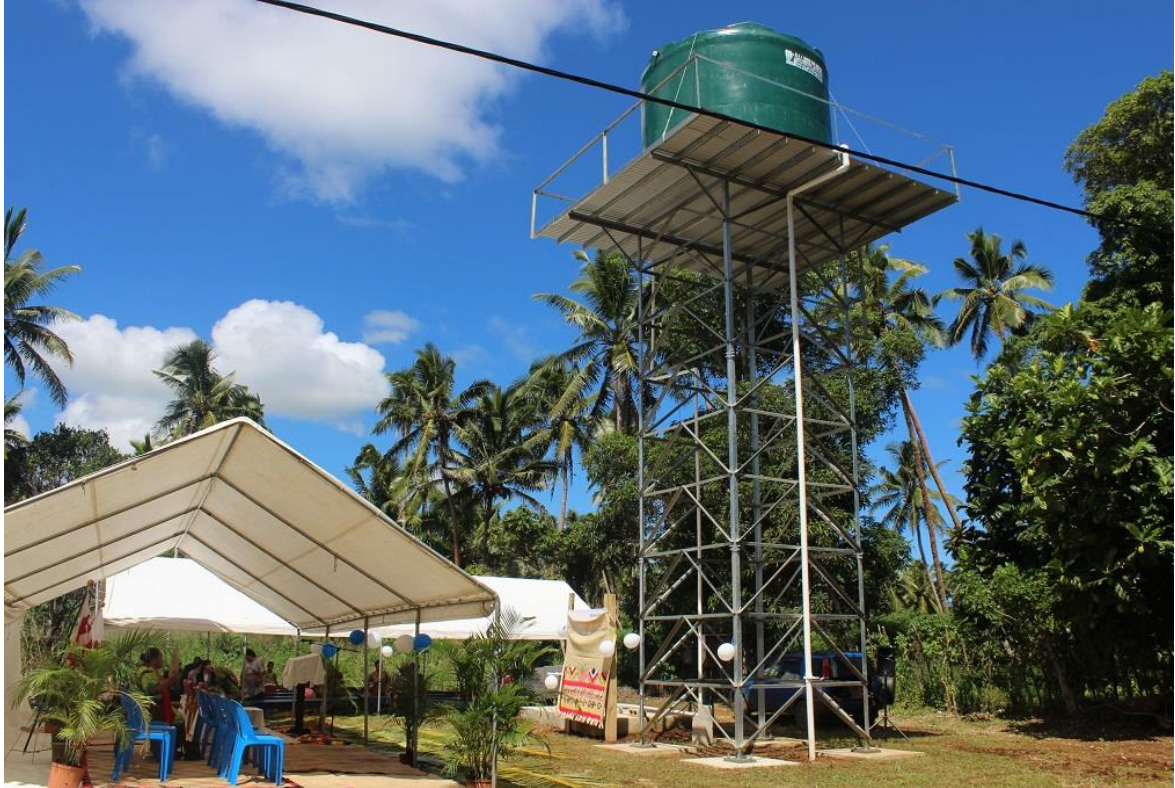
The new water tank and tank stand installed at the western water supply facility of Nukunuku village. .
