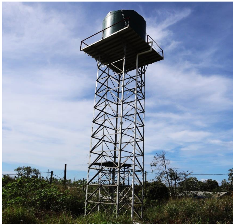
The new 12m tank stand for Vaini village water committee no.1
